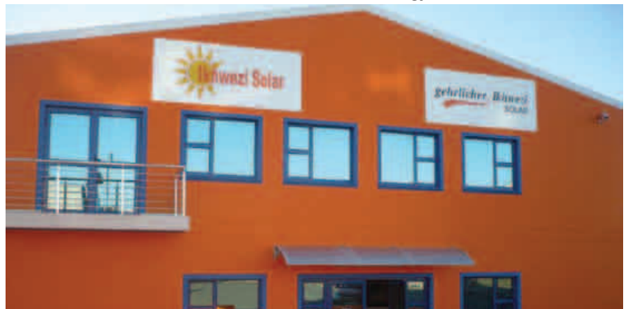
Offices of Ikwezi Solar located in the East London IDZ
